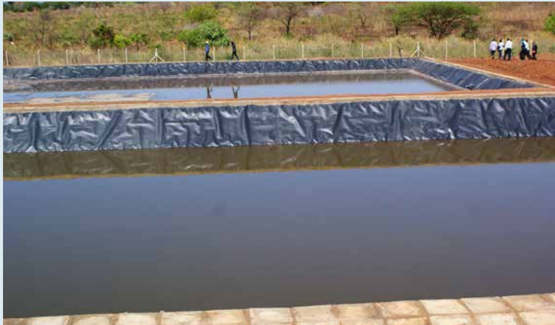
(Above) The artificial wetland; (Below) The facultative and maturation pond. Photos: AMREF
