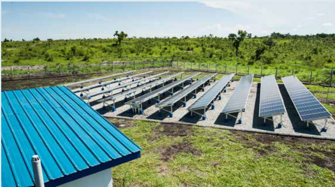
DRC Rhino 50000 ltr per hour solar powered water system . Photo: DRC
