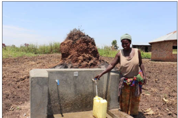
Below, a beneficiary collects water from the installed piped water system
