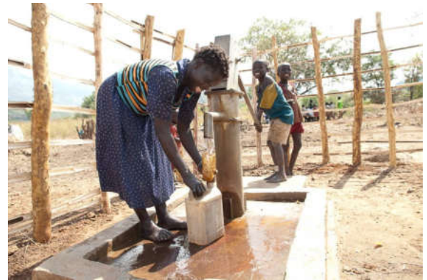
A community member accessing water. Photo by Lifewater International
