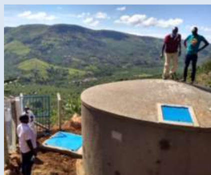
The 30,000 Litre reservoir tank - serves the upper line
