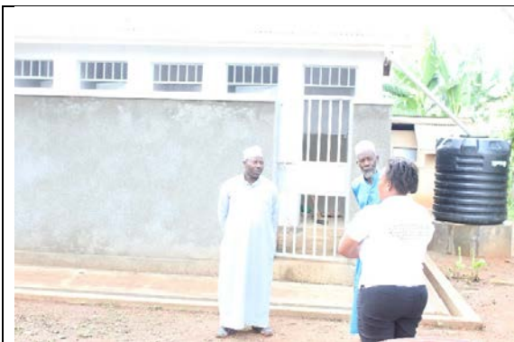
Figure 9; Left to Right, the Headmaster of Kimenyedde, PTA member, and UWASNET staff at the newly constructed toilet block in Kimenyedde
