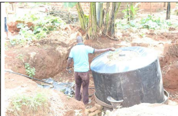
Figure 10; Newly constructed Biodigester
