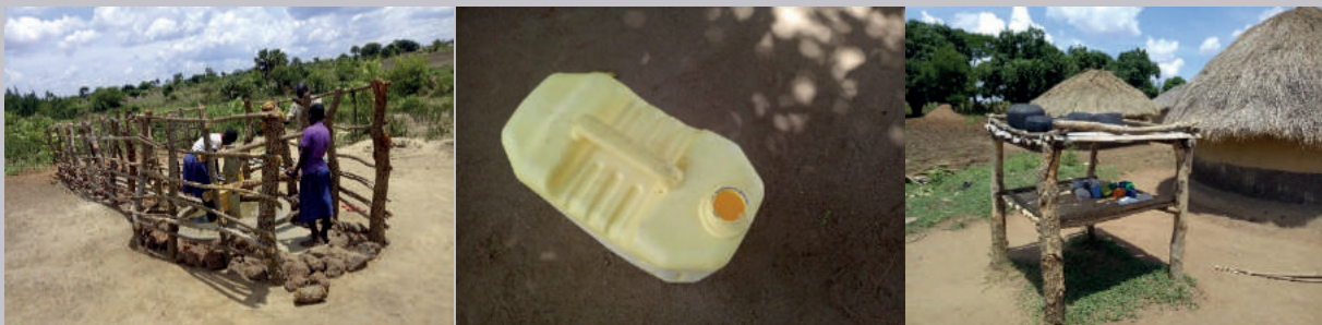
Figure 2: The newly constructed borehole and other sanitation facilities as a result of the project at Okoldyang village
