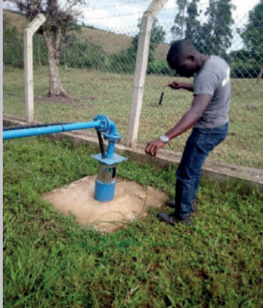
Installation of the diver in the well
